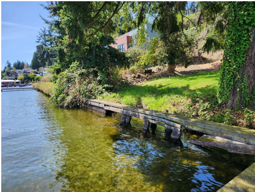
Figure 2. Existing condition of timber bulkhead.
